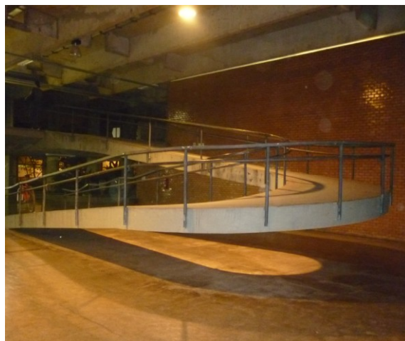
Figura 2.6 – Rampa do ICC UnB.
