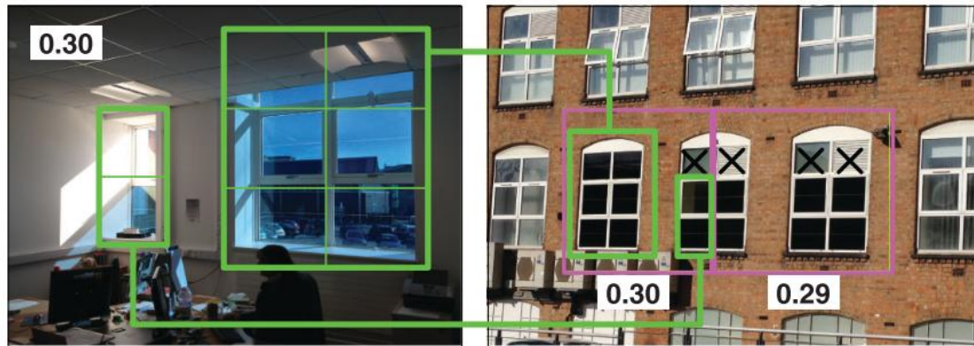
Figure 19 - Photograph of the room equipped with electrochromic glazing at Montford University in Leicester, United Kingdom ( 52^{\circ} north/ 1.1^{\circ} east).
