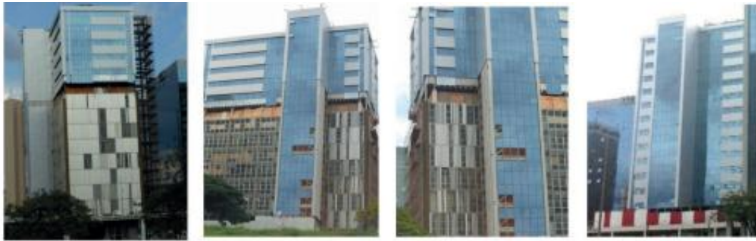
Figure 8 – Chronology of the facade intervention of a building in Brasilia – Setor Comercial Sul: replacement of the brise-soleil to reflective glasses.
