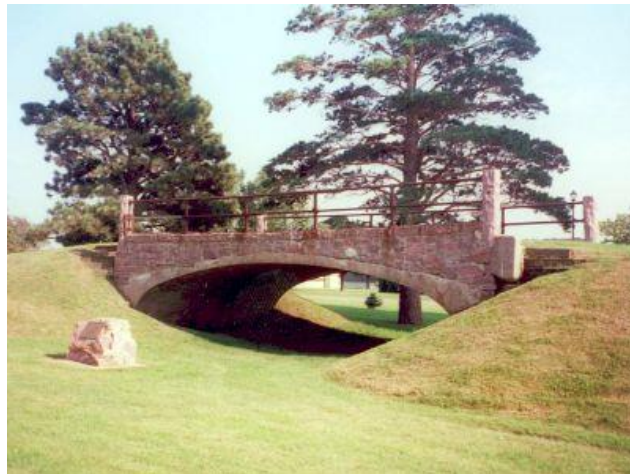
Figura 2.1- Rock Rapids Bridge (SMITH, 2013).
