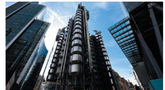
Figura 46 – Lloyd Building, Richard Rogers, 1986.
