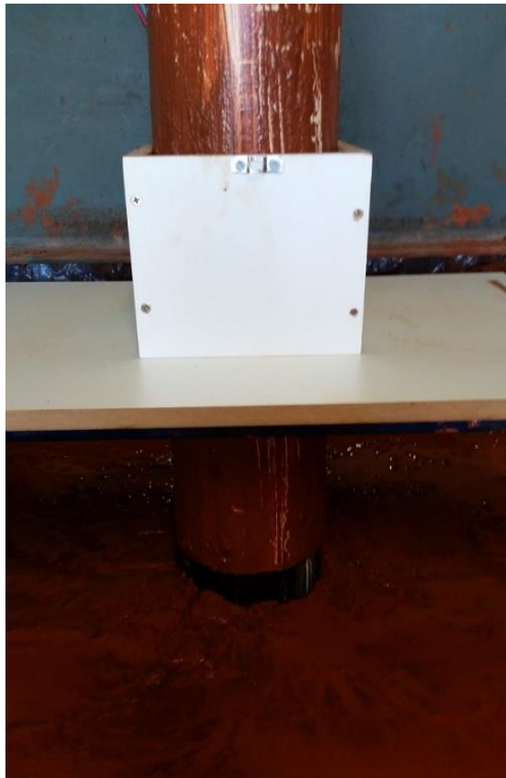
Figure 3.16. Use of the wood casing for pipe insertion.
