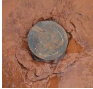
Figure 3.32. Footing area of the loading tests.
