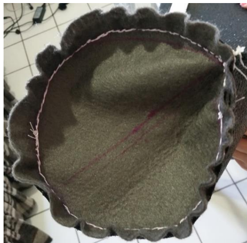
Figure 3.5. Use of non-woven geotextile to seal the bottom of encasement.
