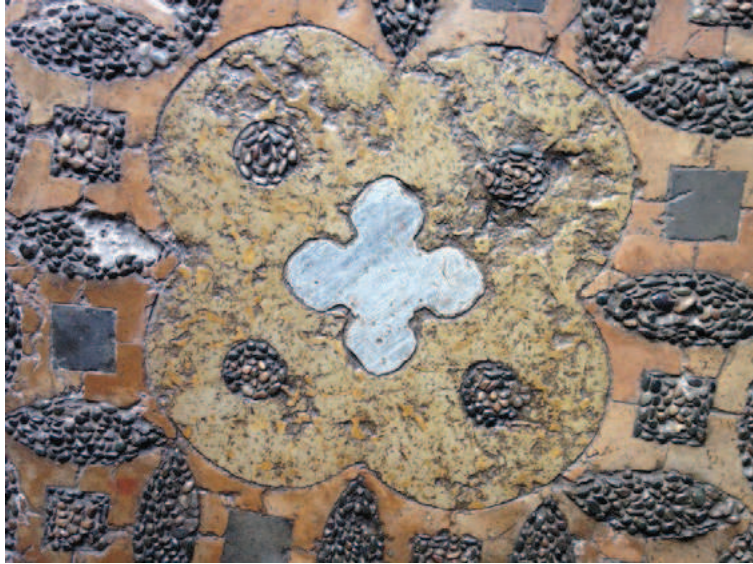
Photograph 4 Example of restoration service – Paving with stones. Author: Marco Aurélio da Silva Máximo
