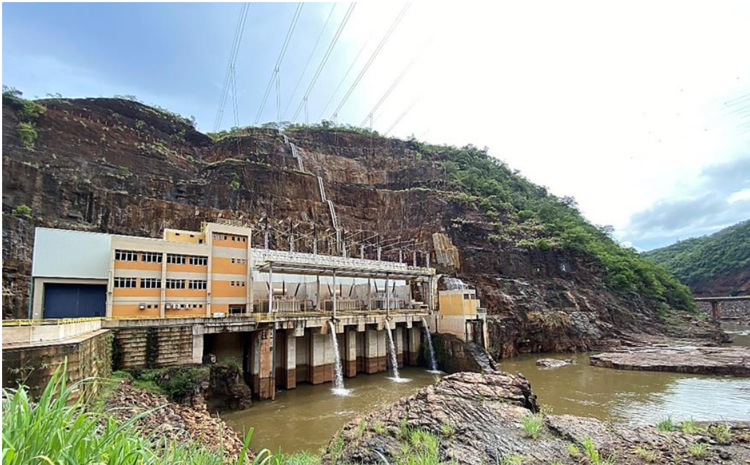
Figure 3.2. Photo of Irapé Hydroelectric power plant surrounded by mica-schist rocks, photo taken during the fieldwork.
