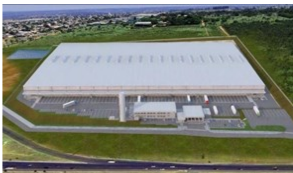
Figura 17 - XP Exeter II Brasília Distribution Center
