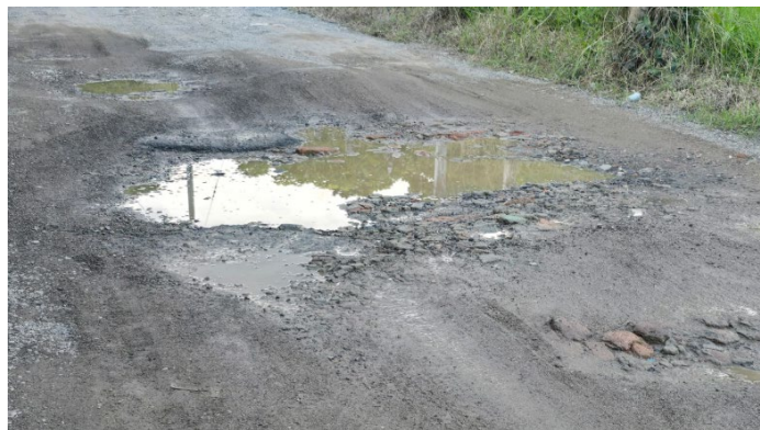
Figure 2.18 - Potholes on unpaved roads.
