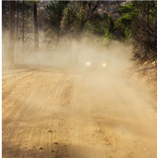
Figure 2.15 - Excessive dust on unpaved roads (Retrieved from https://jethrojeff.com/ ).
