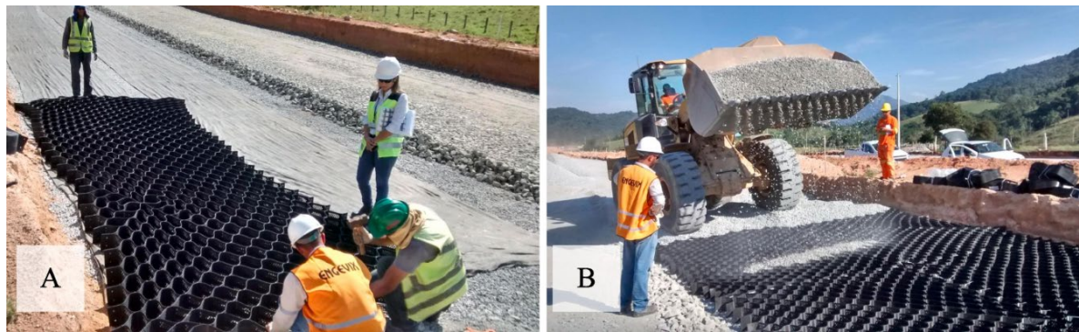
Figure 2.1- Example of geocell installation in the field: (A) Installation. (B) Filling of the geocells.(Feng et al., 2024).
