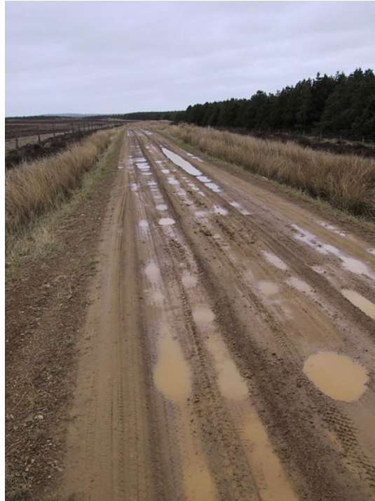
Figure 2.17 - Rutting on unpaved roads (Retrieved from https://www.roadex.org/e-learning/lessons/permanent-deformation/permanent-deformation-rutting-classification/ ).
