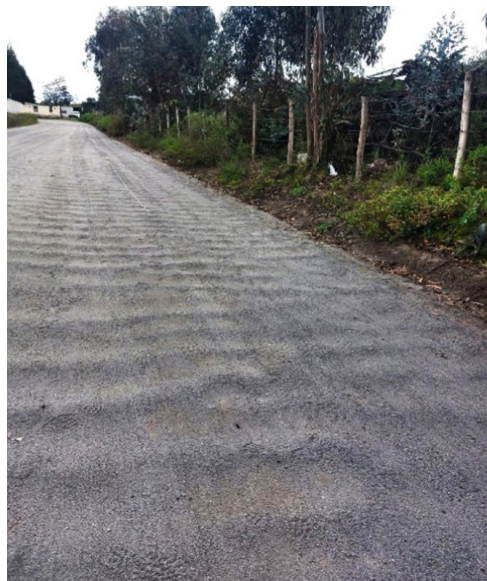
Figure 2.16 - Ondulations on unpaved roads (Ibagón et al., 2025).
