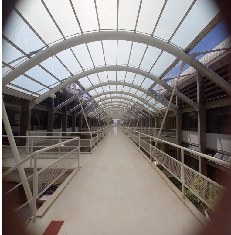
Figure 2: Structure of the Chemistry Building – IQ/UNB
