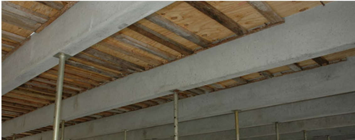
Figure 3: Photo of concrete beams.
