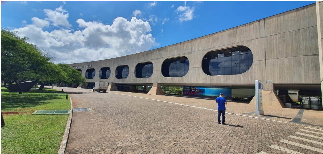
Figure 1 – View of the external wall of the Tancredo Neves building showing the openings and the columns, shaped as pyramid trunks.
