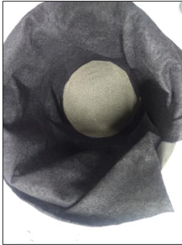
Figure 3.18. Placement of geotextile and the bottom sand layer.
