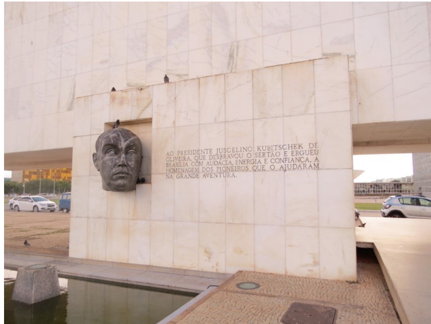
Fig. 7: City Museum, detail of the East Facade. Source: Eduardo Oliveira Soares, 2017.
