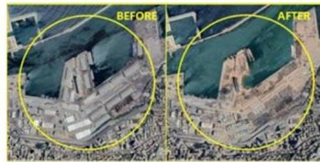
Figure 1: Images before and after the explosion at the Beirut Port. As you can see, everything was destroyed in a radius of 400 m from the explosion point.
