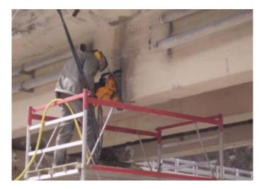
Figure 21 – View of artificial introduction of damage in longitudinal beam.
