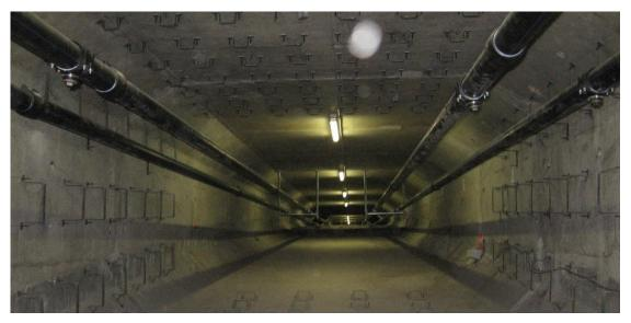
Figure 9. General view of the external prestressing cables installed in the bridge deck.
