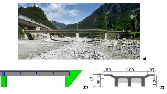
Figure 12 – Picture with overview of Dogna Bridge (a) and its schematic representation of longitudinal view (b) and transversal section (c).
