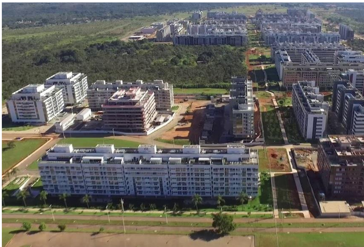
Figure 1: Northwest Sector in Brasília (Brazil). A small green upper left) still remain among the buildings that dominate the former indigenous reserve.
