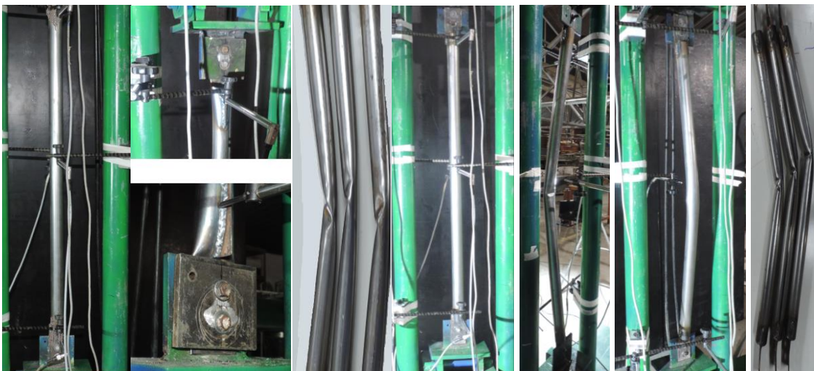
(s) Colapso do BCR1175 com \lambda = 90
