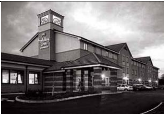
Figura 2. 38 – Hotel na Inglaterra ( http://www.steel-sci.org/lightsteel )
