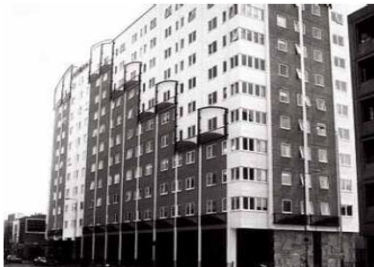
Figura 2.44 – Reforma de fachada usando steel frame ( http://www.steel-sci.org/lightsteel )
