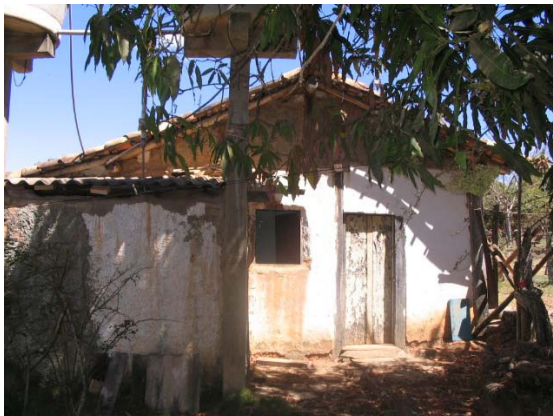
Figura 250 – Fachada lateral (Acervo PROAU/FAU/UnB).
