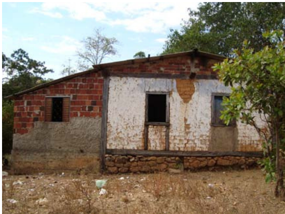
Figura 130 – Fachada lateral (Acervo PROAU/FAU/UnB).
