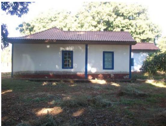
Figura 274 – Fachada lateral (Acervo PROAU/FAU/UnB).
