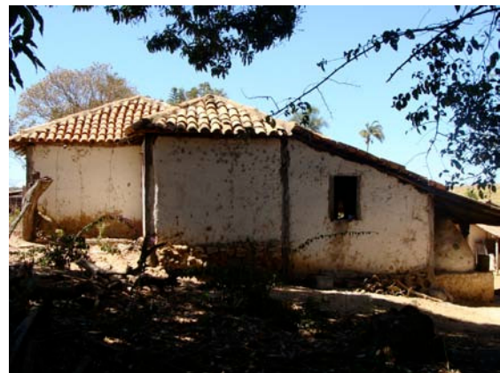
Figura 231 – Fachada lateral (Acervo PROAU/FAU/UnB).
