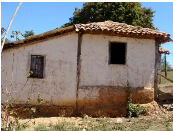
Figura 230 – Fachada lateral (Acervo PROAU/FAU/UnB).
