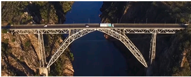
Fig. 2. Dom Pedro II steel bridge with 237 m of span with a height of 86 m over San Francisco River in Brazil.
