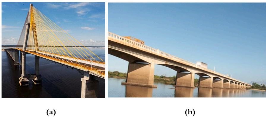
Fig. 3. (a) The Biggest cable-stayed Bridge in Brazil pass over the Rio Negro, has a central span of 400 m with a mast of 185.00 m of high; (b) Felipe Guerra Bridge over the Piranhas/Açu River with 585 m of extension with 2 main beams of section variable type parabolic.
