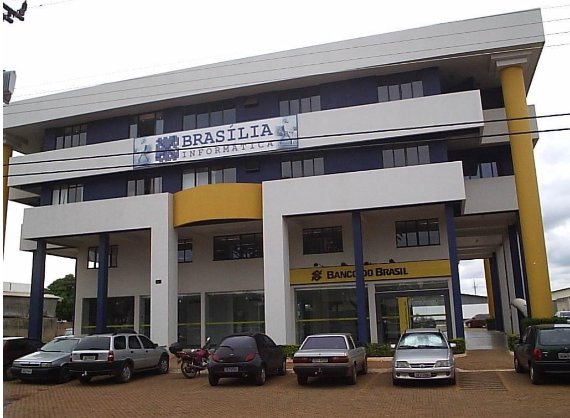
Figure 1 – Main façade of the studied building, during the first inspection in 2005.
