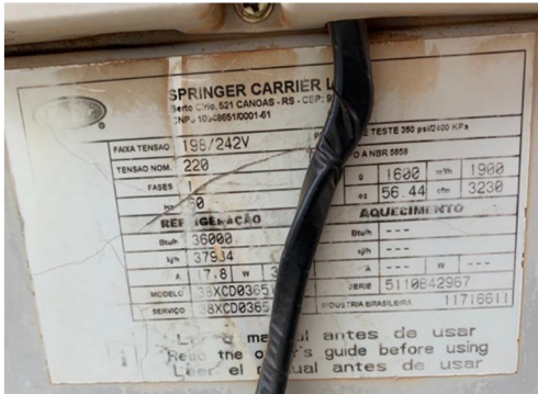
Fig. 10. Technical specifications of the air conditioning units in the building
