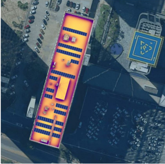
Fig. 26. Shading areas at the photovoltaic system
