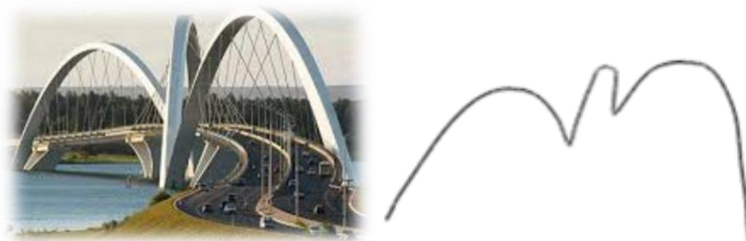
Figure 2 - JK Bridge and initial profile
